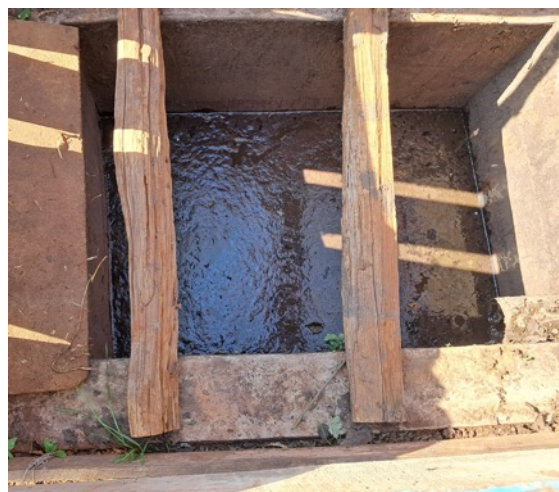
Slurry concrete pit
