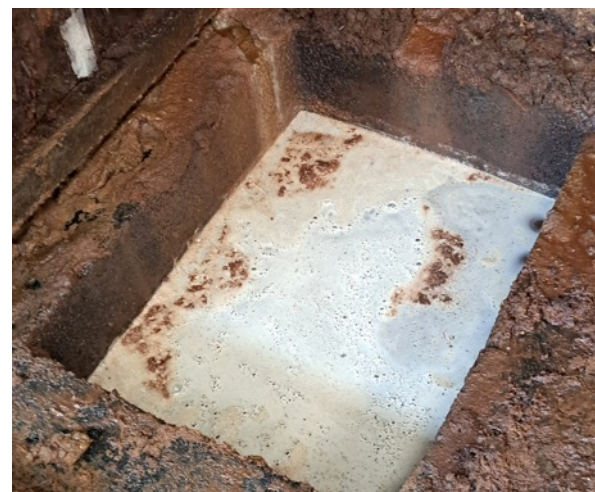
Urine concrete pit
